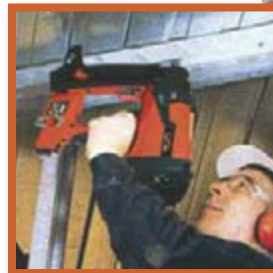
● Drywall track fixing onto steel
