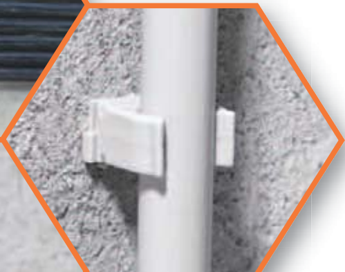
● Electrical conduit saddle fixing
