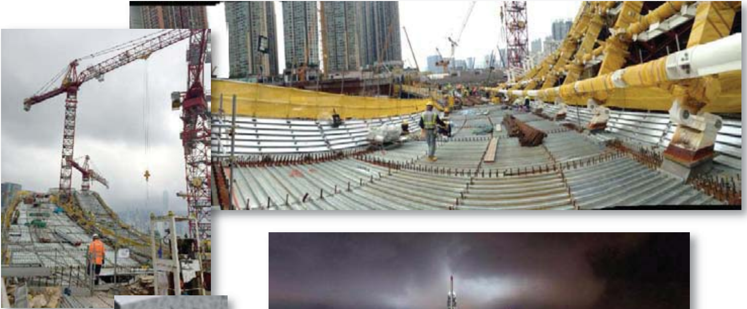
● Steel decking fixing onto beam
