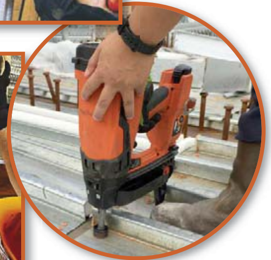
● Wall tie bracket fixing
