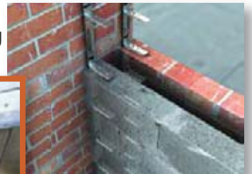
● Wall tie bracket fixing
