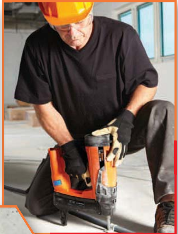
● Electrical conduit saddle fixing
