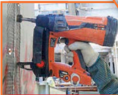
● Wire mesh fixing onto steel column
