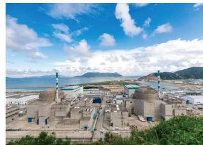
Guohuapan Power EPC Project
