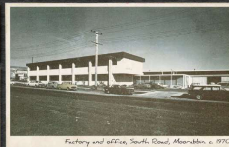
Factory and office, South Road, Moorabbin c.1970
